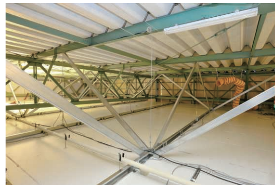
NEQRES® quakeproof ceilings were developed after the Great East Japan Earthquake. None of the ceilings fell during the 2016 Kumamoto earthquakes.
