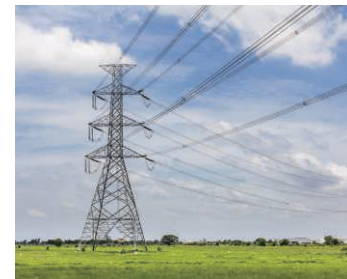
Overhead electric lines and a steel tower
