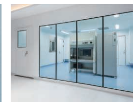
A clean room using flat panels
